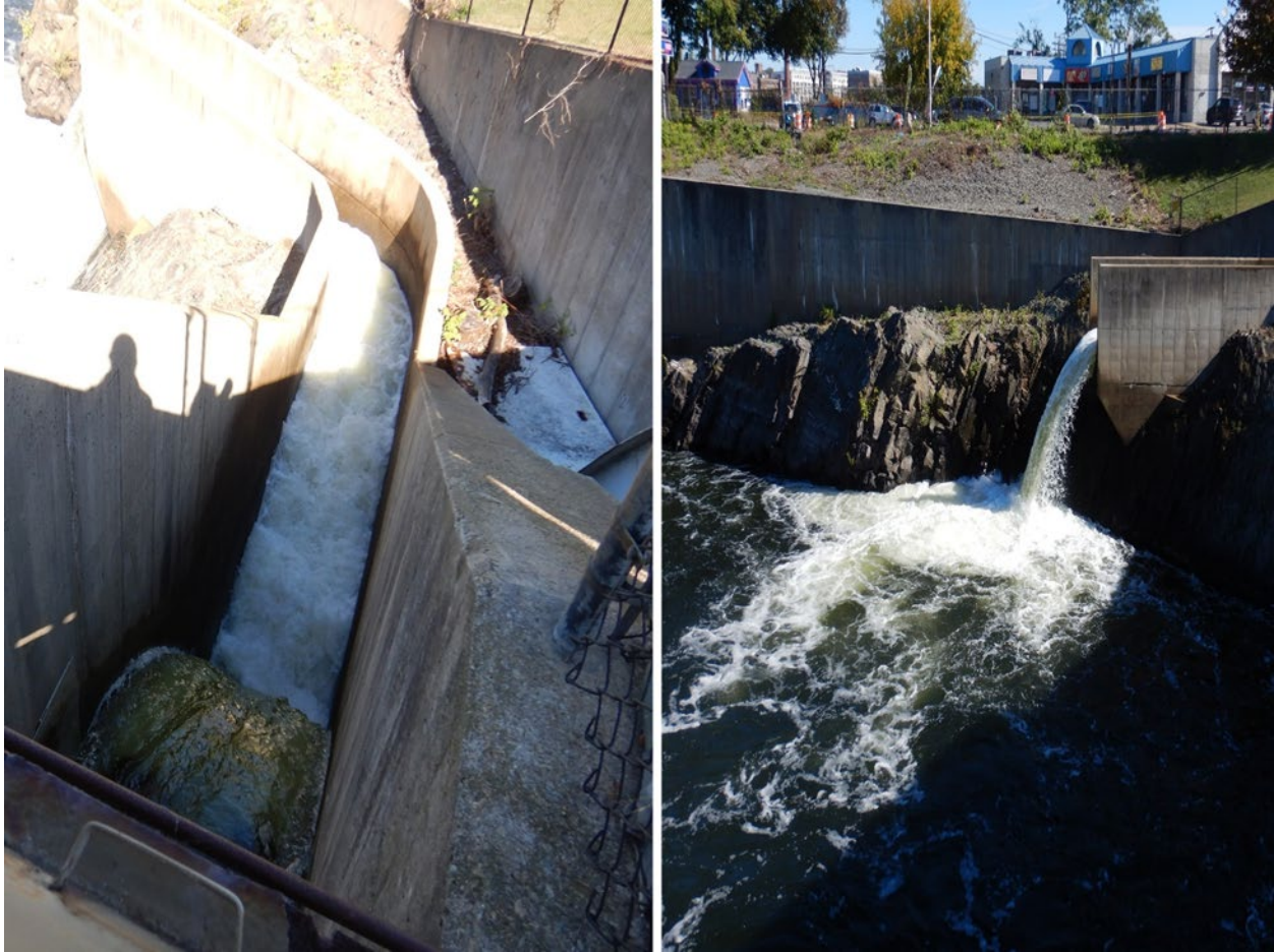
Figure 2-1 Downstream bypass conditions during the 2025 Downstream Juvenile Alosine Passage Assessment. Upstream plunge (left image) and tailrace plunge (right image) show conditions representing typical discharge (160 cfs).
