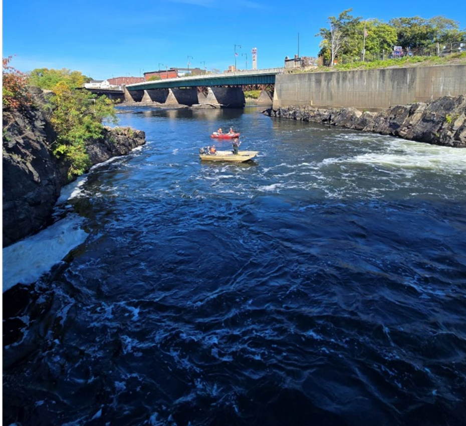
Figure 4-6. Recapture boats in the tailrace of Lawrence Hydroelectric Project.
