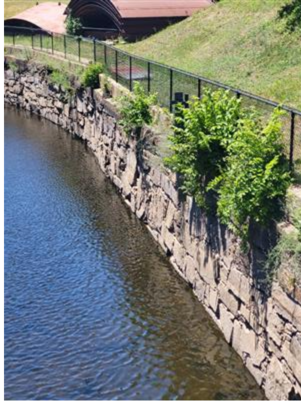
Photo 18: Representative photo of tree-of-heaven, Lawrence Hydroelectric South Canal, June 28 th , 2024.
