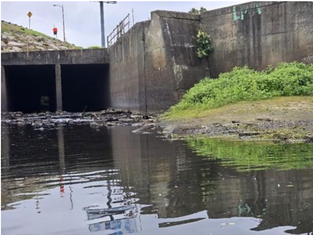
Photo 36. Bank vegetation at Study location T31 downstream of the wingwall.
