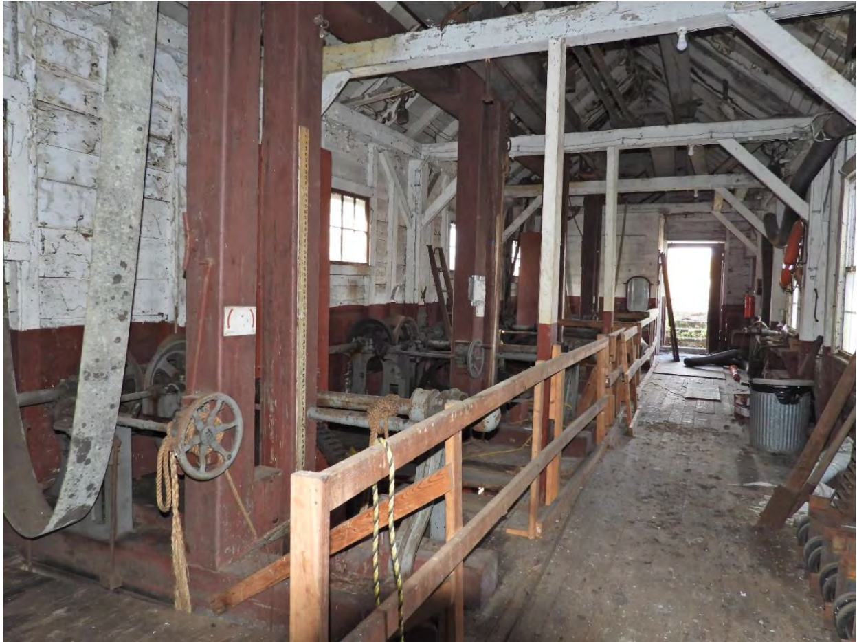
Figure 6-25. Interior view of the South Canal Gatehouse, showing gate arrangement and gate-lifting equipment; view facing northwest.
