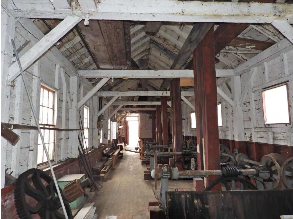
Figure 6-8. Interior view of the North Canal Gatehouse, showing gate arrangement and gate-lifting equipment; view facing southeast.
