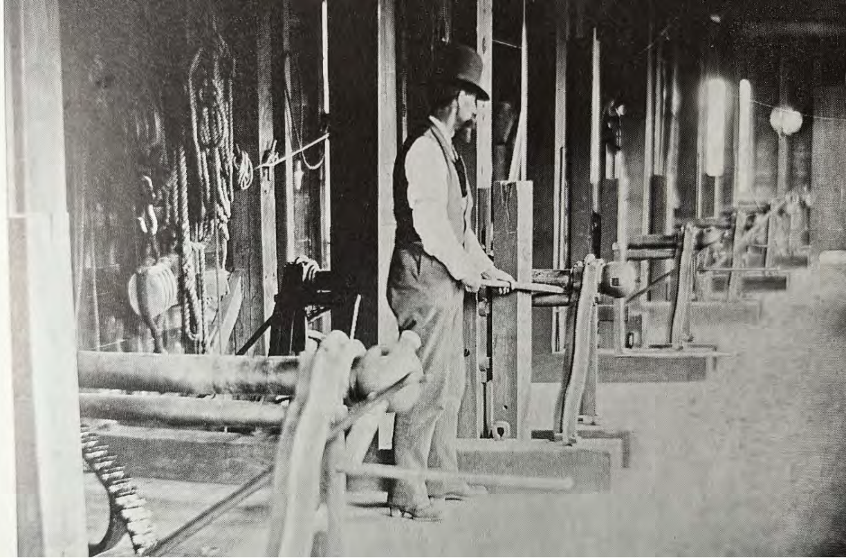
Figure 6-12. Interior view of the North Canal Gatehouse in 1898, showing gate tender Tom Holmes operating a gate.
