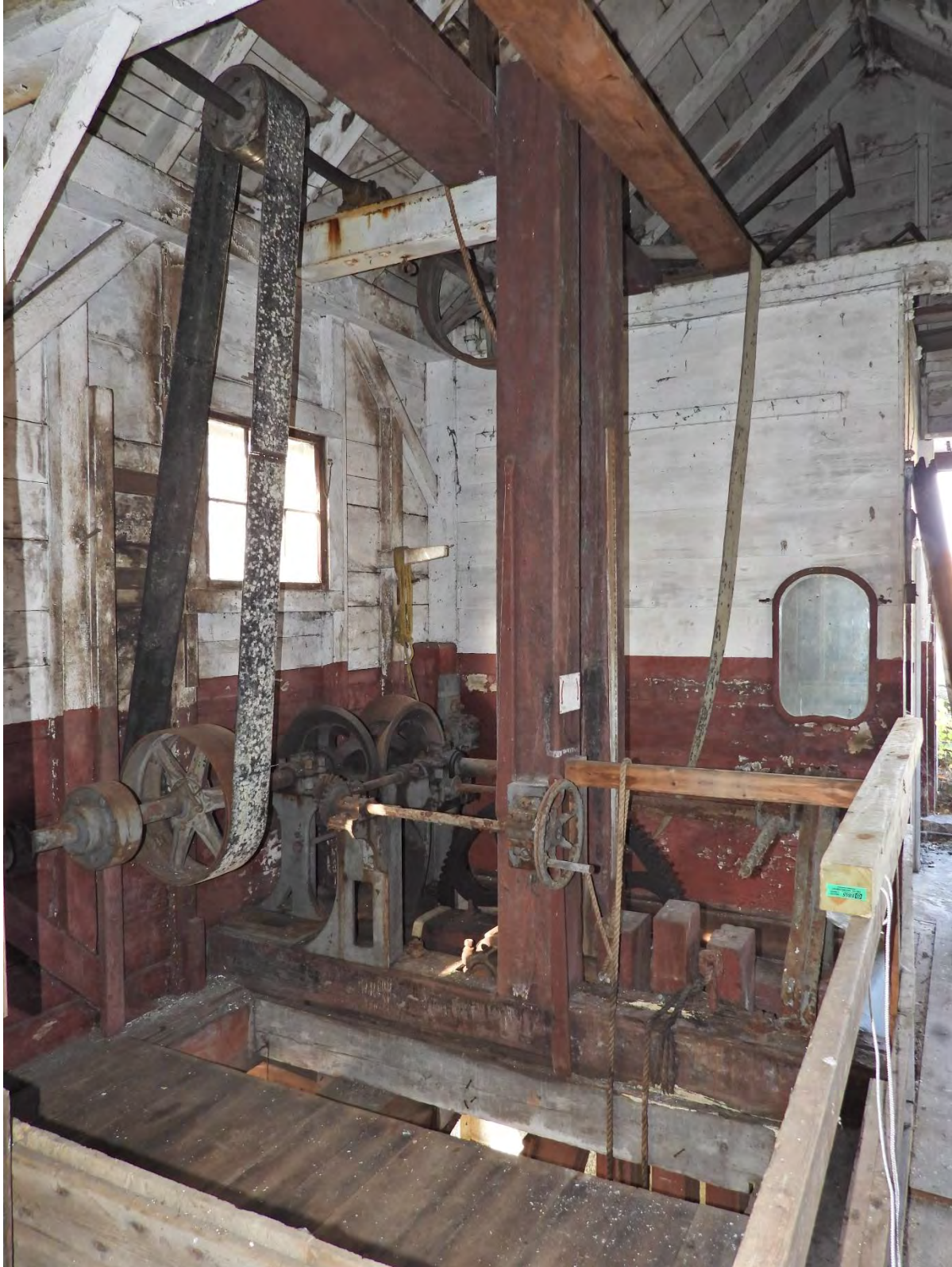
Figure 6-27. Detail of the South Canal Gatehouse manual and electric hoisting systems, view facing west.
