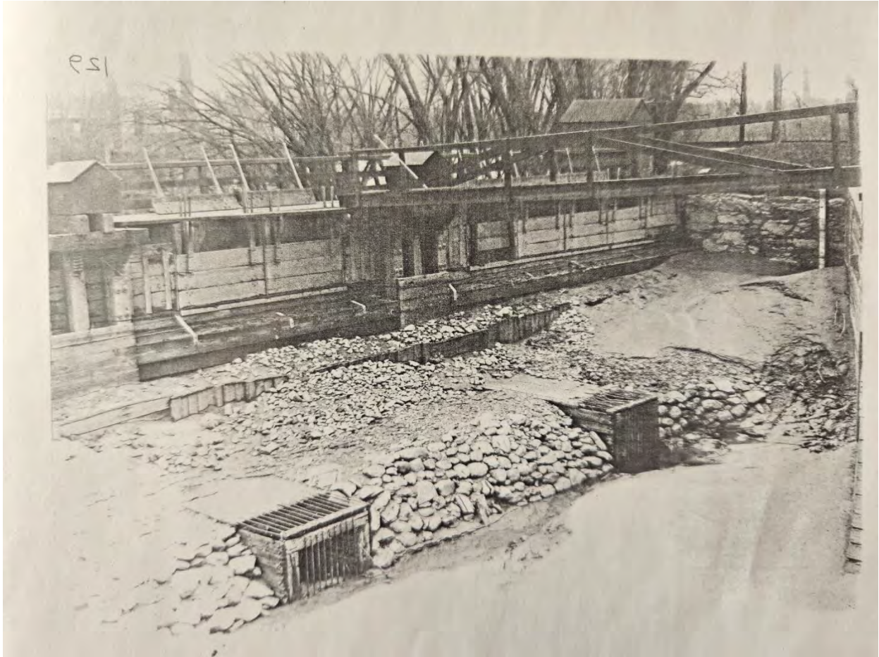
Figure 6-18. Undated photograph of the North Canal Wasteway, showing upstream view of drains and their hoist enclosures.
