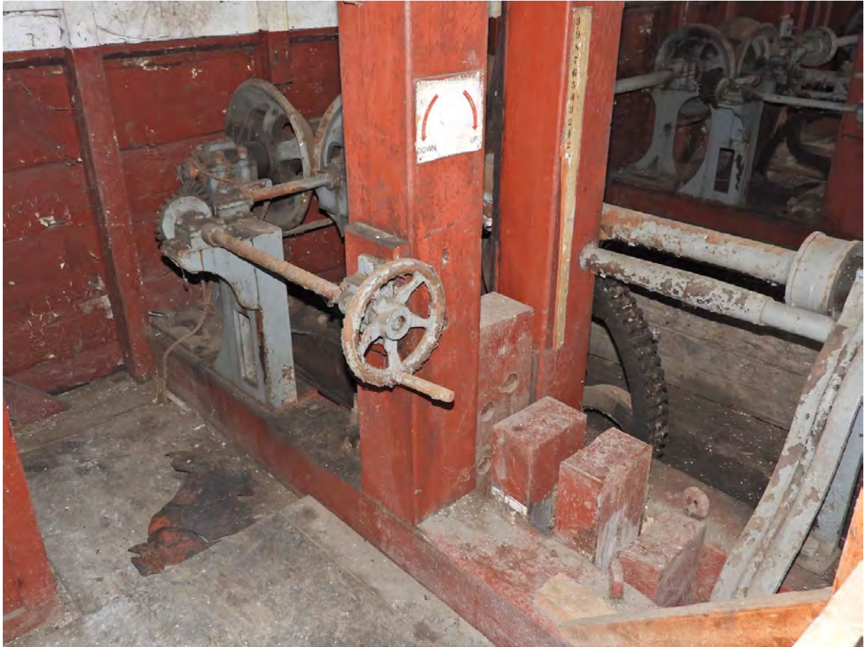
Figure 6-9. Detail of the North Canal Gatehouse gate hoist, with leaf gate stems visible on the lower right; view facing northwest.
