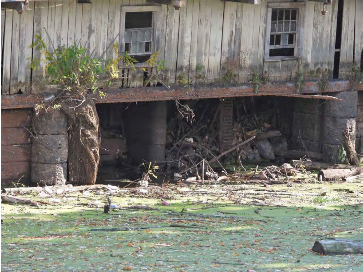
Figure 6-4. Upstream image of the North Canal Gatehouse showing the two open middle sluiceways and a single gate stem.
