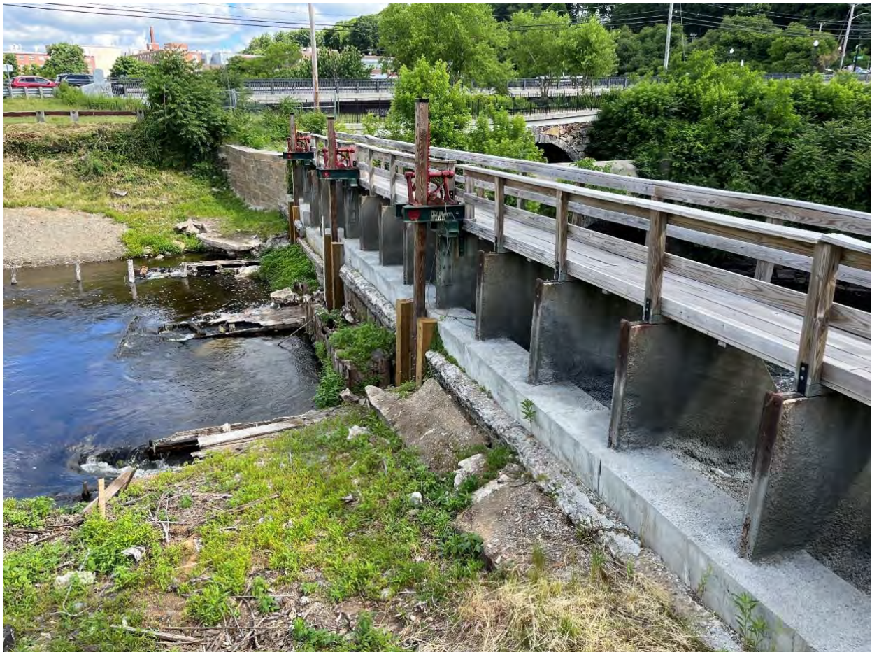
Figure 6-14. Upstream view of the North Canal Wasteway with sluiceways and drain gate hoists, view facing north.
