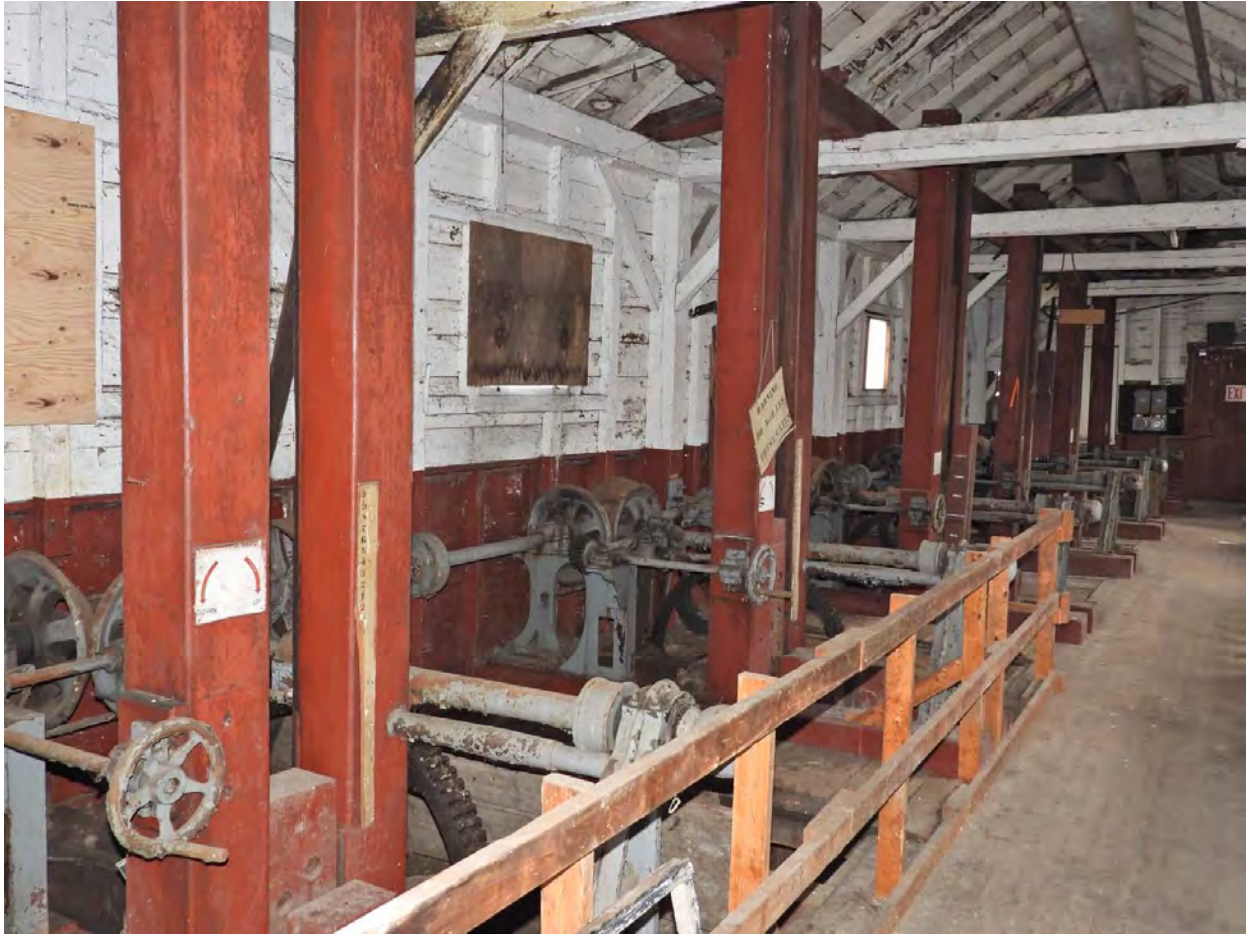
Figure 6-7. Interior view of the North Canal Gatehouse, showing gate arrangement and gate-lifting equipment; view facing northwest.
