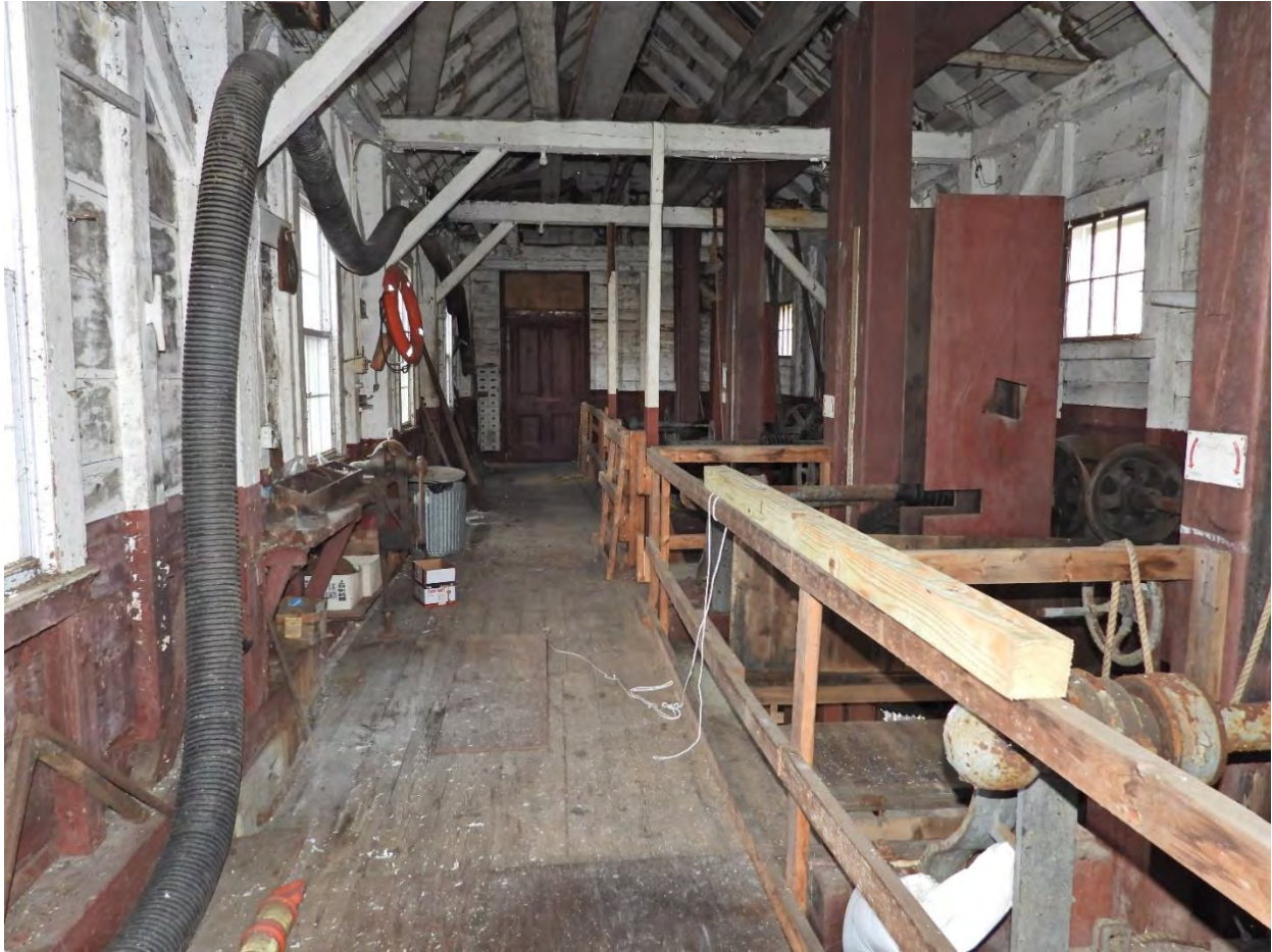
Figure 6-26. Interior view of the South Canal Gatehouse, showing gate arrangement and gate-lifting equipment; view facing southeast.
