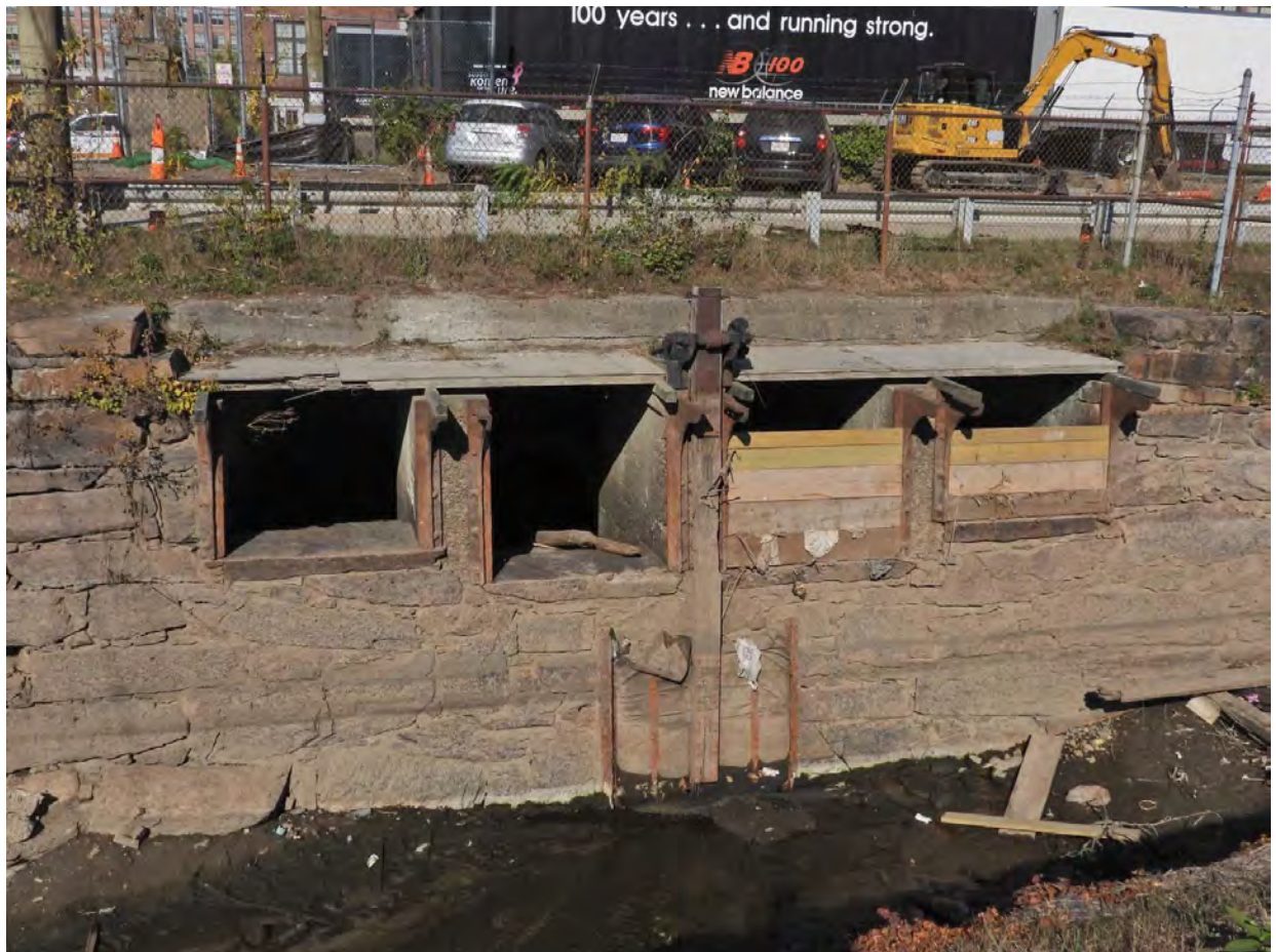
Figure 6-34. View of the South Canal Wasteway with sluiceways, flashboards, drain gate, and hoist; view facing northwest.
