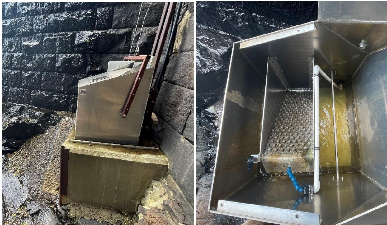
Figure 3-2. North side eel lift approach substrate and collection hopper (left photo) and cast aluminum climbing substrate and water supply in the hopper (right photo).
