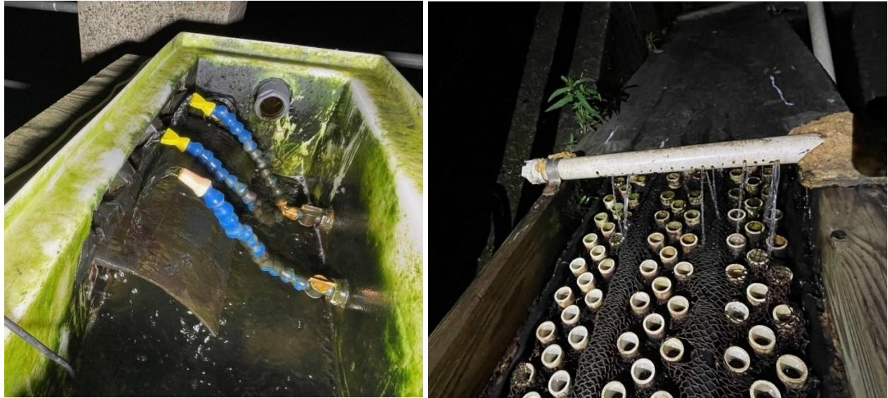
Figure 5-2. View of the south side eel trap collection tank (left photo) and ramp (right photo) water supply during the July 25, 2024 survey.
