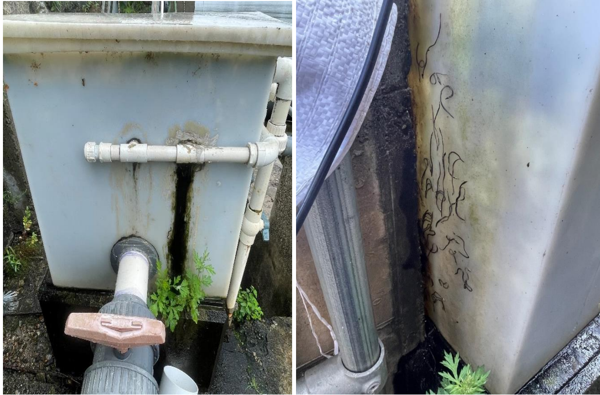
Figure 5-6. Dried algal growth (left photo) and desiccated juvenile eels (right photo) left in areas of previously observed leakage flows associated with the south side eel trap collection tank.
