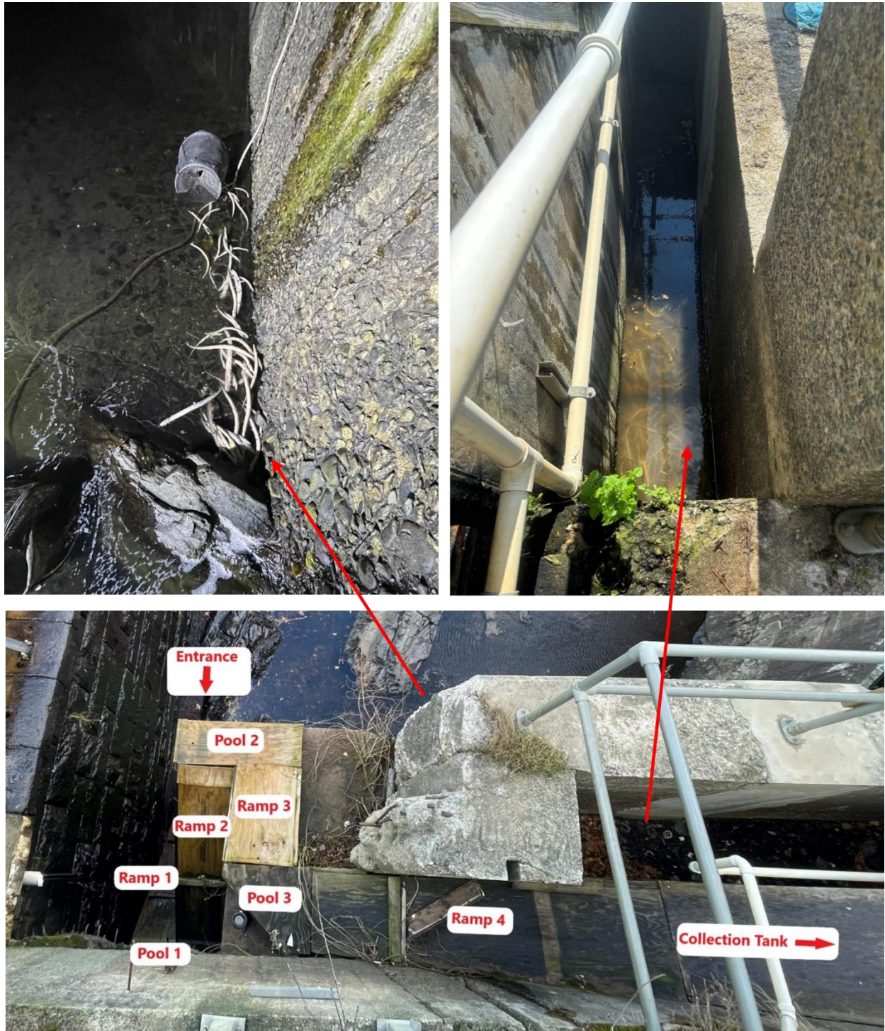
Figure 5-5. Juvenile eel mortality areas associated with the south side eel ramp observed during July at the base of trough leakage (left photo) and inside the trough adjacent ramp section 4 (right photo).
