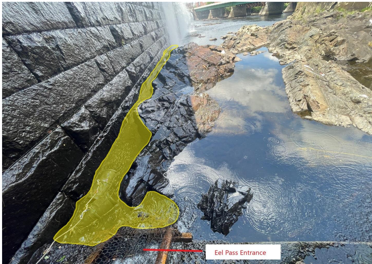
Figure 5-1. View of the south side eel trap entrance and the approach pools conveying attraction water to the Lawrence tailrace.
